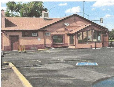
Front of the Chapter 3 Building.
